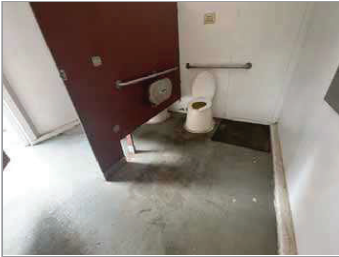
TOILET STALL OVERVIEW
