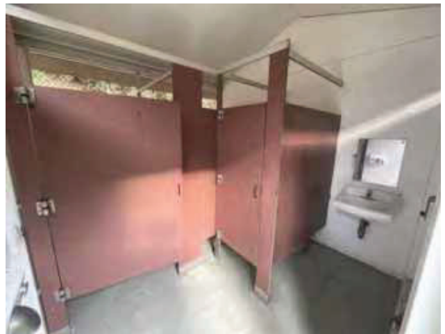
6 - RESTROOMS INTERIOR OVERVIEW
