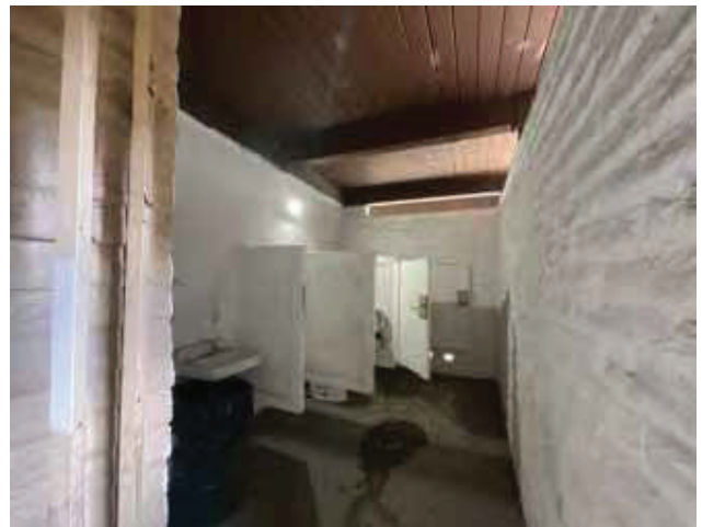
6 - RESTROOMS BUILDING INTERIOR
