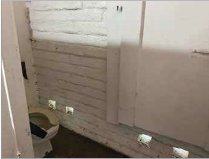
TOILET STALL OVERVIEW
