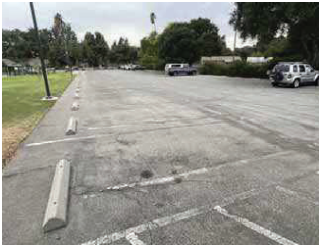
3 - OVERVIEW EAST TO WEST
