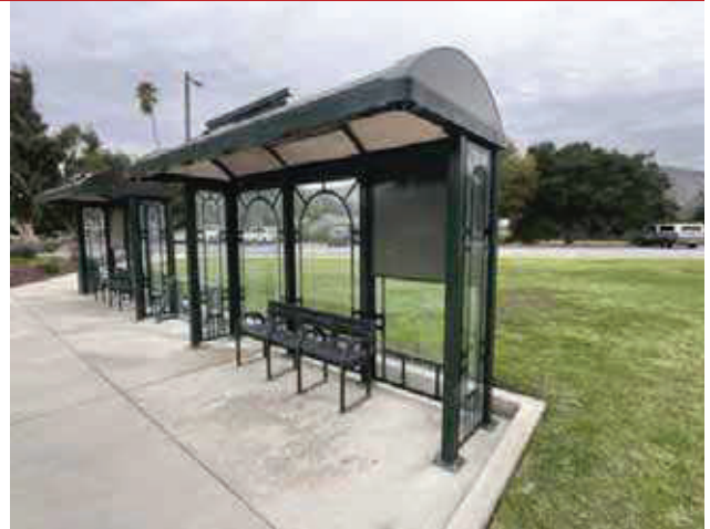
8 - BUS STOP SHADE STRUCTURE
