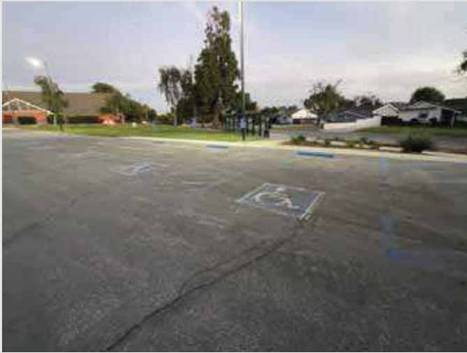
OVERVIEW OF ACCESSIBLE PARKING AREA
