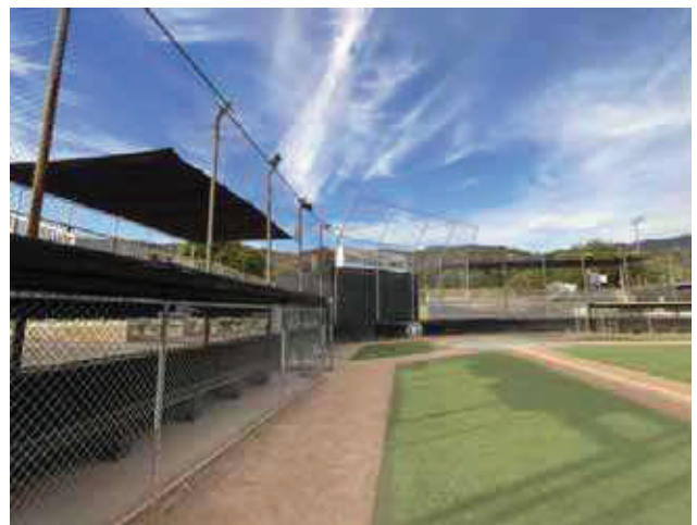
6 - BACKSTOP CHAIN-LINK FENCE
