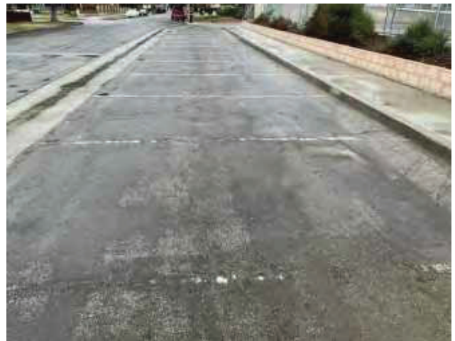
6 - WEST PARKING LOT
