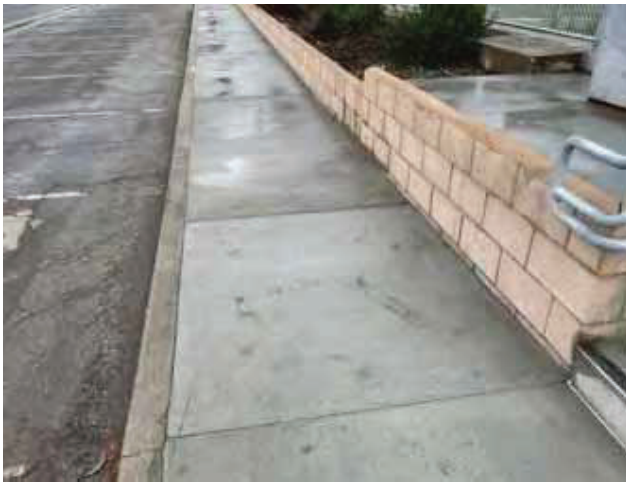
9 - SMALL CONCRETE SIDEWALK
