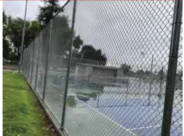
14 - CHAIN LINK FENCE
