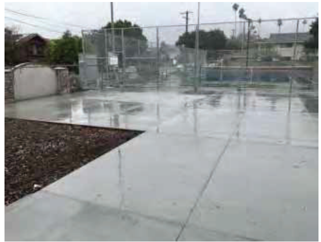
10 - LARGE CONCRETE SIDEWALK
