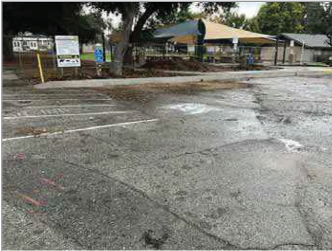
OVERVIEW OF ACCESSIBLE PARKING AREA
