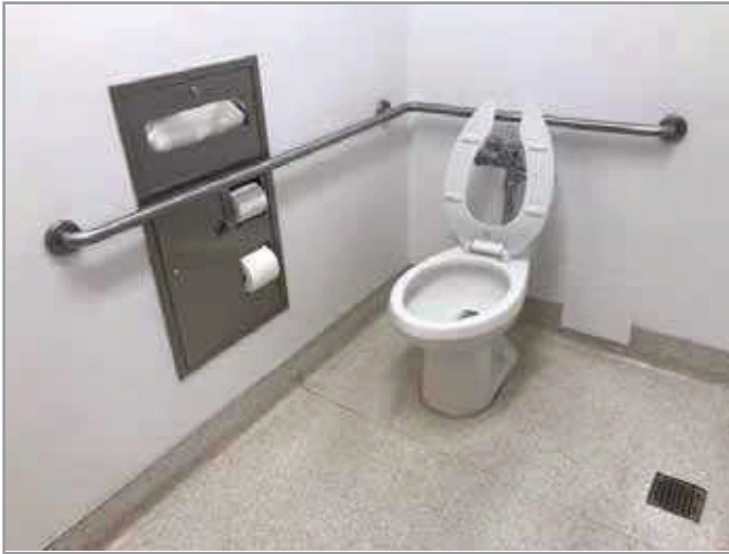
TOILET STALL OVERVIEW
