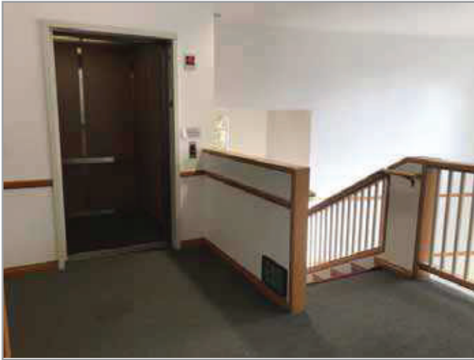
LOBBY LOOKING AT CABS (WITH DOORS OPEN)
