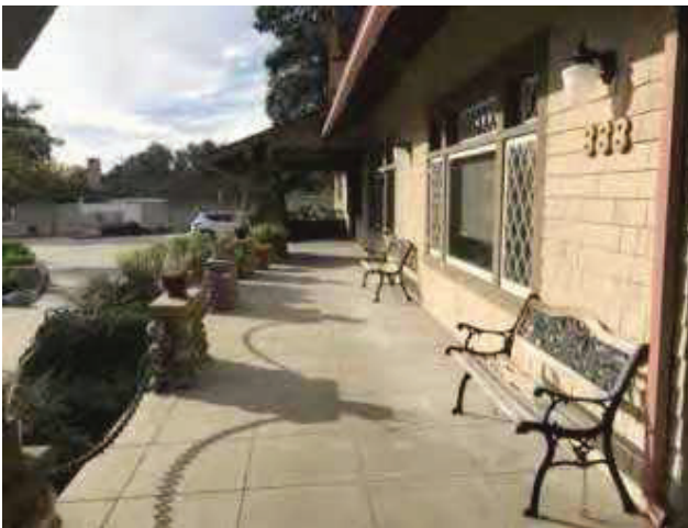
23 - CONCRETE PAVED PATIO AREA
