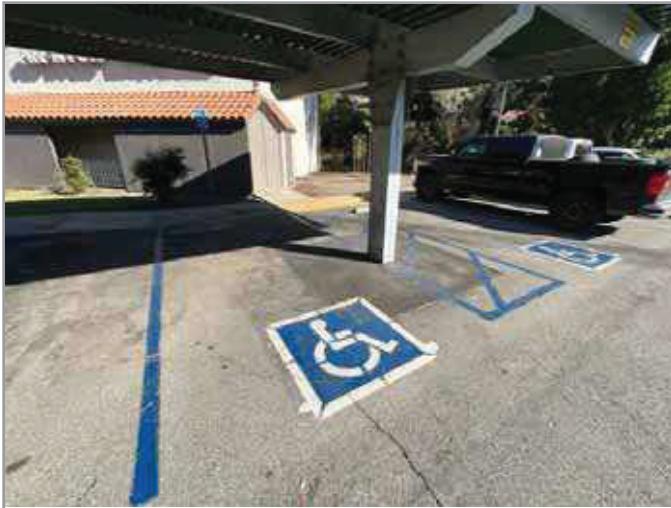
OVERVIEW OF ACCESSIBLE PARKING AREA
