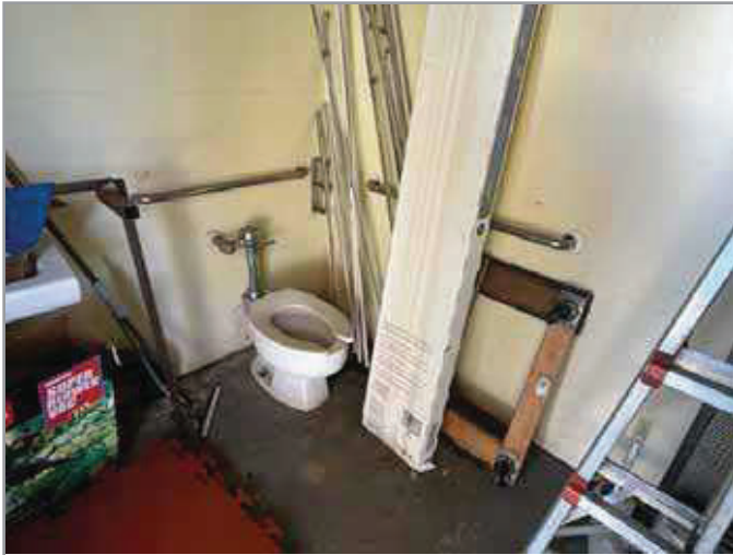
TOILET STALL OVERVIEW
