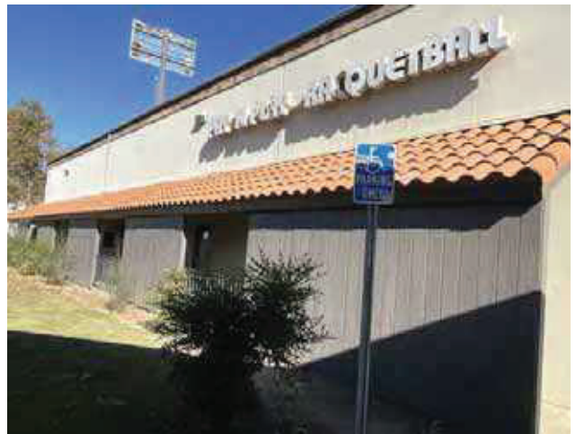
6 - CLAY TILE ROOFING
