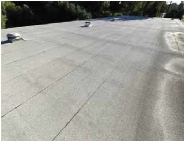
5 - MODIFIED BITUMEN ROOFING
