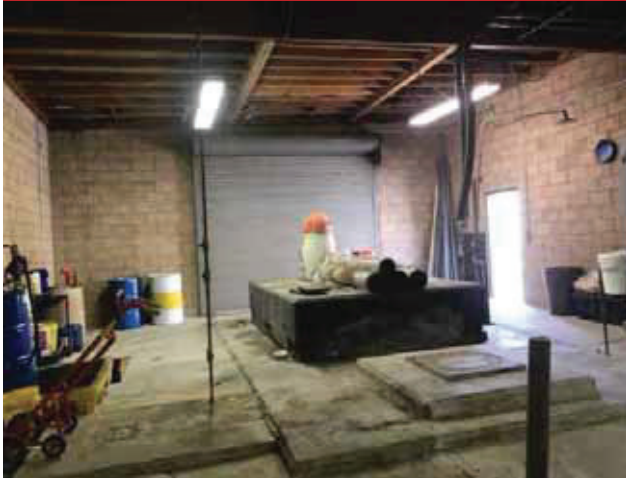
19 - STORAGE BUILDING INTERIOR AREA
