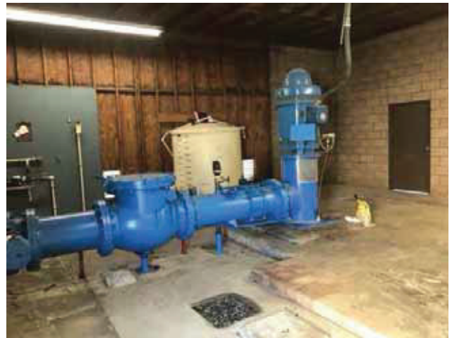
16 - WELL BUILDING NO.12E INTERIOR
