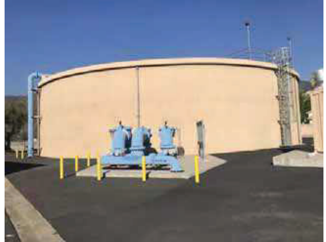
26 - WATER RESERVOIR CONCRETE STRUCTURE
