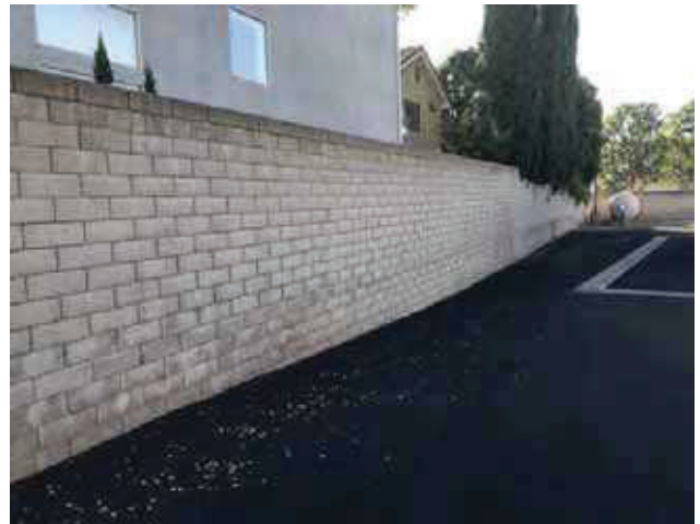
28 - CMU WALL SITE FENCING
