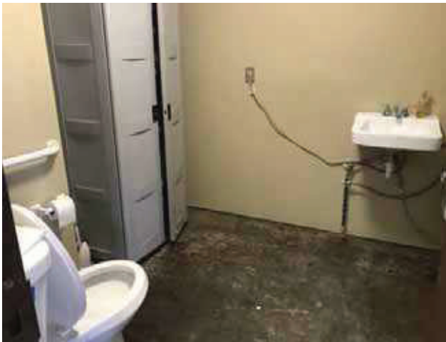
15 - TYPICAL STAFF RESTROOM INTERIOR
