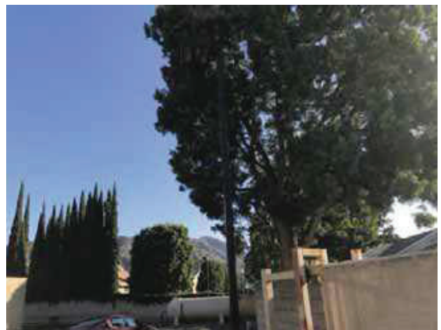
30 - SITE AREA POLE LIGHT
