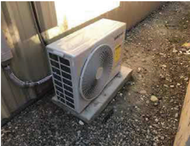
21 - DUCTLESS SPLIT SYSTEM AIR CONDITIONER
