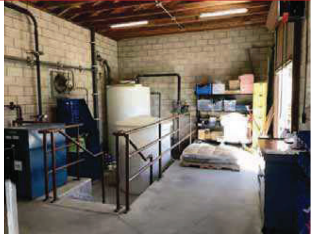
14 - CHEMICAL BUILDING INTERIOR AREA
