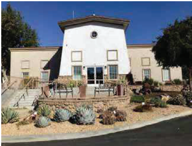
9 - WATER DEPARTMENT OFFICE FRONT ELEVATION
