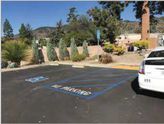
OVERVIEW OF ACCESSIBLE PARKING AREA
