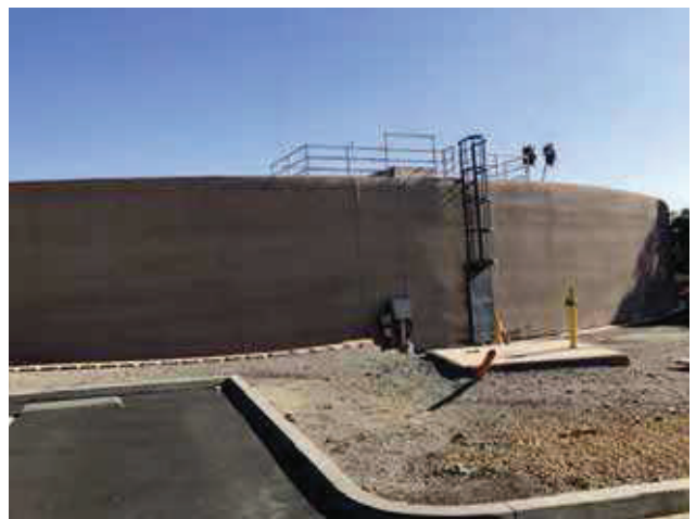
30 - WATER RESERVOIR CONCRETE STRUCTURE
