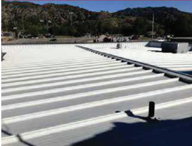
13 - WATER DEPARTMENT METAL ROOFING
