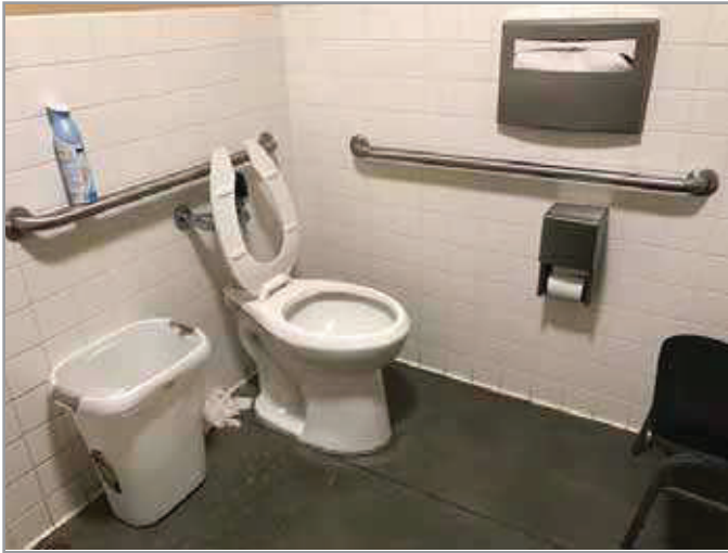
TOILET STALL OVERVIEW
